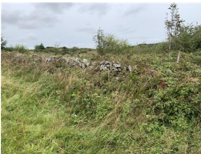
Plate 6.9 Drystone wall (BL1) at field boundary.
