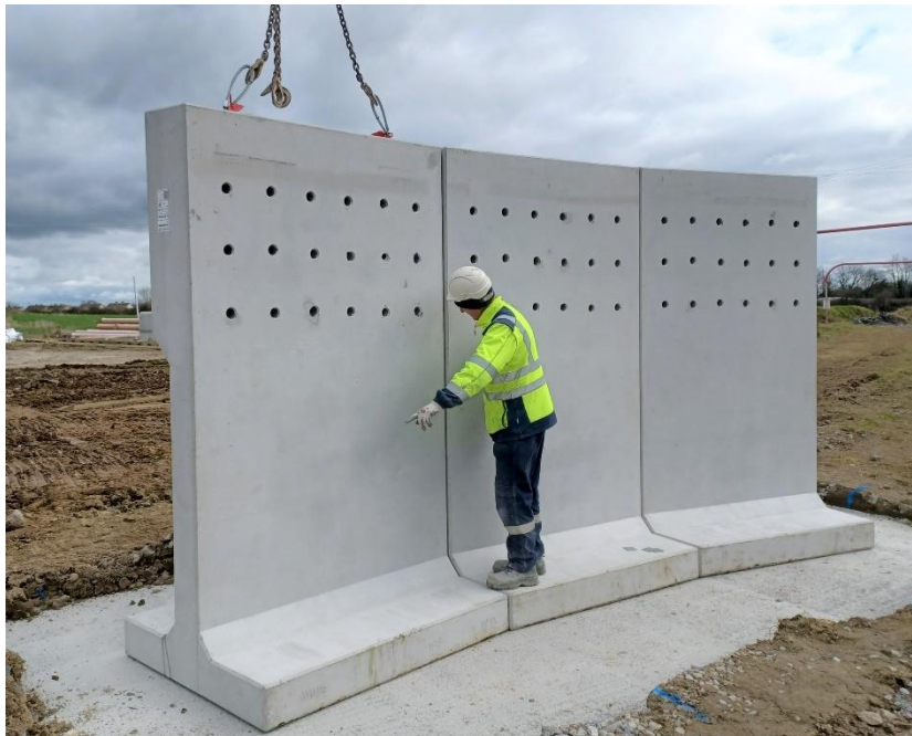
Plate 6.16 Pre-cast Sand Martin nesting wall.
